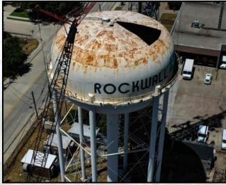
It will take approximately 30 days to dismantle the water tower. The process includes using a cutting torch to cut the water tower into smaller pieces and lowering them to the ground, working from the top down. Watch for regular updates and pictures of the process as it happens.
